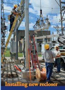
**Above** Corn Belt Power's electrical maintentance and transmission crews install a new recloser at the Hampton Substation Aug. 17 in preparation for the co-op's new Tesla battery system.
